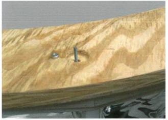
Remove the radius wall from the pallet and move it near the location where it is to be installed. Remove the plywood cap and base. The plywood is held in place with nuts attached to all-thread that extends from the base to the cap. DO NOT REMOVE THE ALL-THREAD, it needs to remain in the wall to help hold the top and bottom frames to the block.
