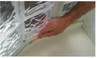
4. Position the radius wall in the exact location where you are going to install it. Make sure you push the wall into the mounting channel snuggly. The mounting channel will accommodate a finished wall that is not plumb. On the finish surface, mark the outline of both sides of the base of the radius wall.
