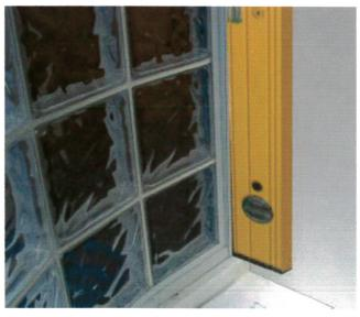
Mark the position of the mounting channel on the finished wall. Make sure that the mounting channel is plumb.
