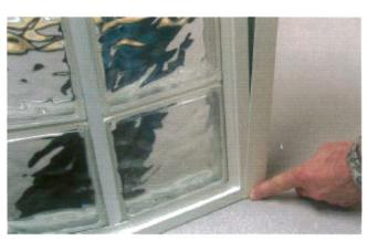
Slip the mounting channel onto the end of the radius wall where it will mount to your finished wall.
