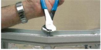
2. Cut the all-thread flush with the top and bottom of the wall.
