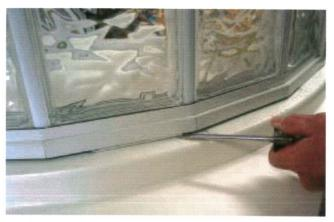
10. Rather than push down the radius wall completely onto the flat caps, use a stiff putty knife or small pry bar to work the flat caps up into the radius wall. Make sure you have the flat caps attached on both sides of the radius.
