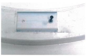
7. Using the outline on the finished surface as a guide, position the pieces of aluminum flat cap with the flanges pointing up. Fasten the caps to the surface with non-corrosive screws and washers. The screws should be snug, but still allow the flat cap to slide with a bit of effort.
