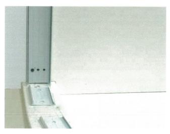
Using the marks on your finished wall, secure the mounting channel to the finished wall.
